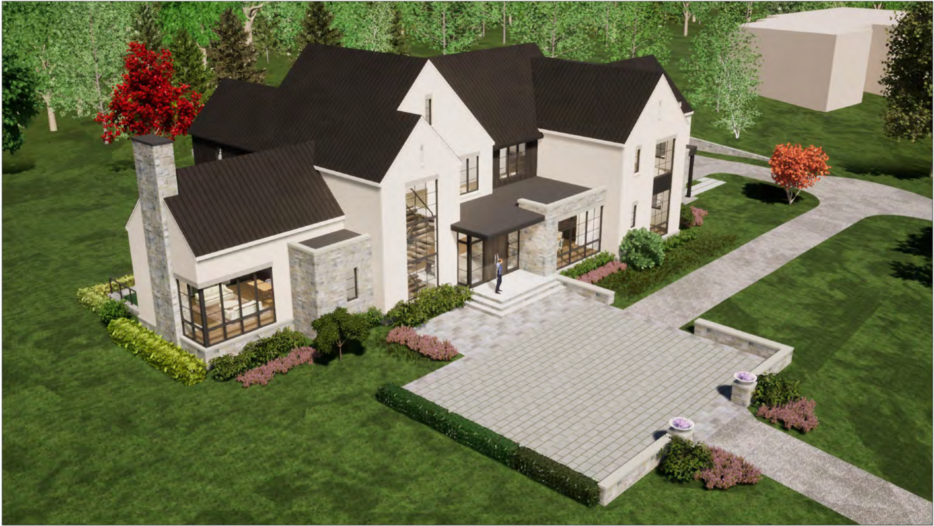
○ AERIAL VIEW FROM THE FRONT AND LEFT SIDE
